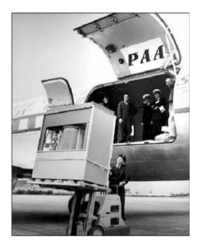
1956 IBM RAMDAC computer included the IBM Model 350 disk storage system
